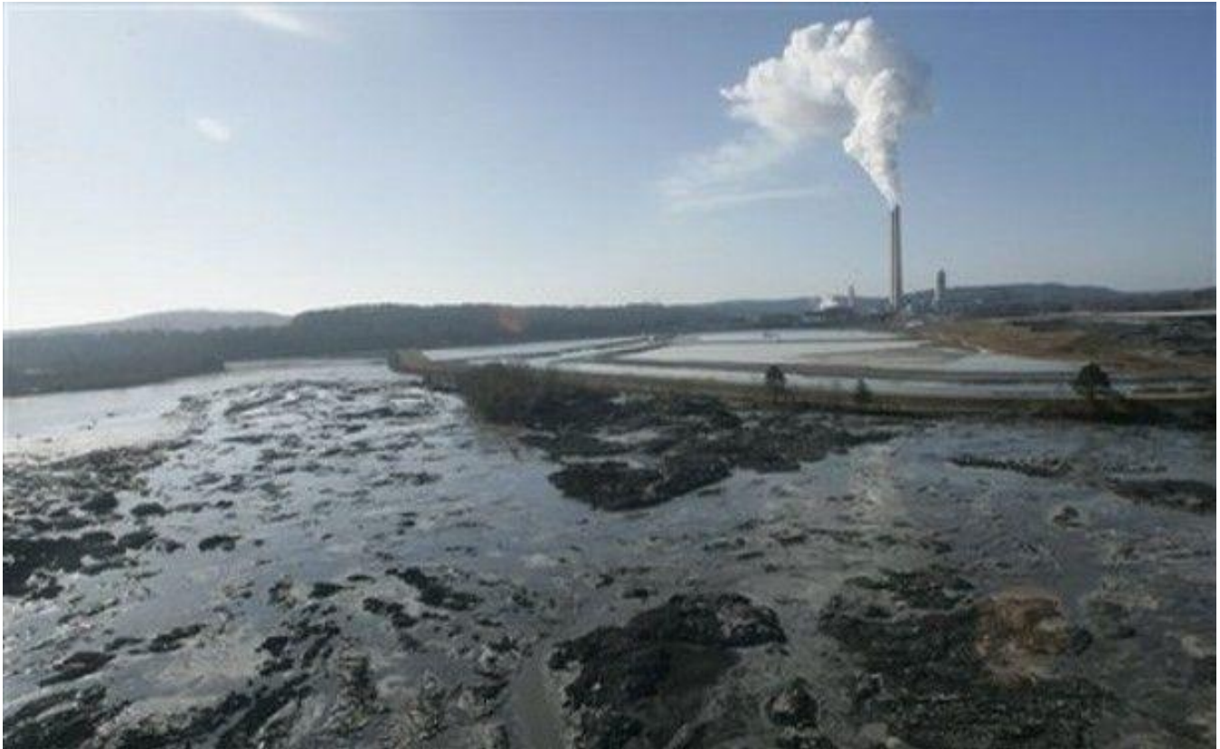
February 19, 2015, Duke coal ash spill sends toxic waste downstream for 70 miles.
